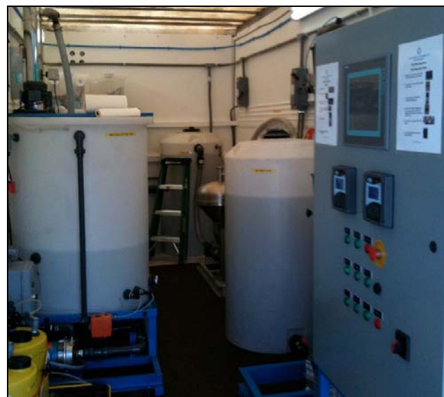
Figure 2. Interior of customized mobile trailer housing CFT Turboclone™ filter and Dow ultrafiltration system.
